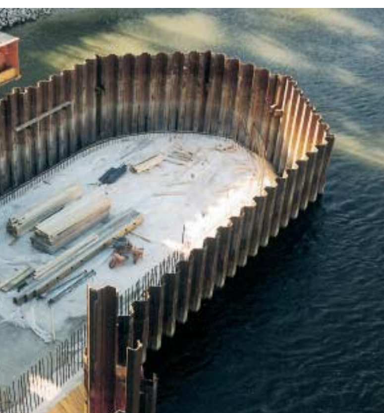
Bridge pier support
