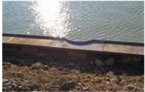
Profiled capping plates are on the top of construction
